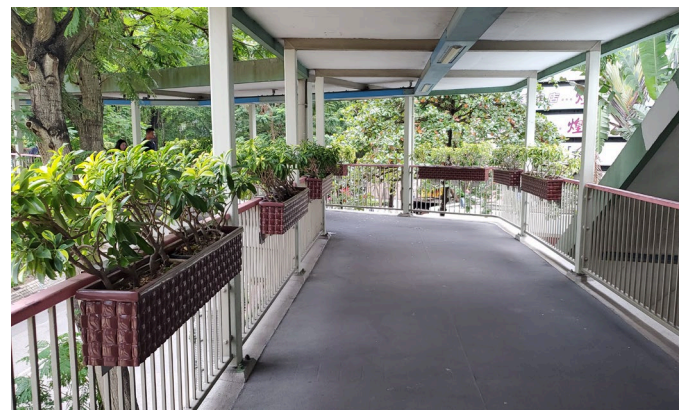
Railing Planters on Footbridge
